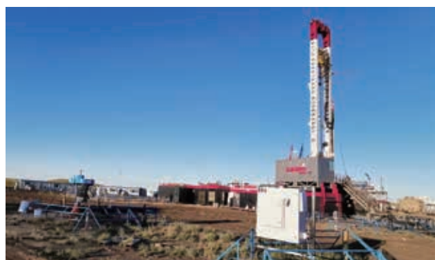
Drilling rig for new wells drilling
