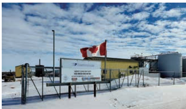
The Group's central battery in Windy Lake region
