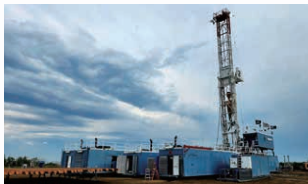
Drilling rig for new wells drilling
